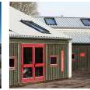
Langebjergh School, Denmark
